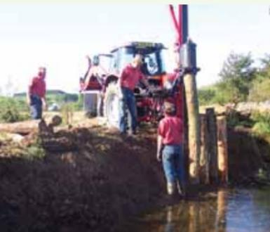
Work underway to install vertical piled timbers as bank protection, Clifton-on-Bowmont, September 2011.
