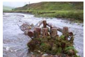
One of the bar apex ELJ features in action on the Swindon Haugh site, demonstrating the capture of sediment material and slowing of flood water flows, September 2012.
