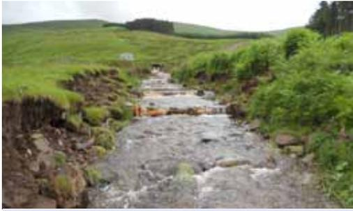
Completed grade control feature on the Kelsocleugh Burn, in the headwaters of the Bowmont catchment, June 2012.
