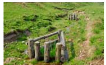
Bar Apex ELJ feature at Kelsocleuch, one of 12 constructed at this site, showing final element of specification – native tree planting within each feature.
