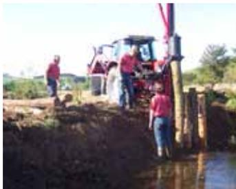
Work underway to install vertical piled timbers as bank protection, Clifton-on-Bowmont, September 2011.
